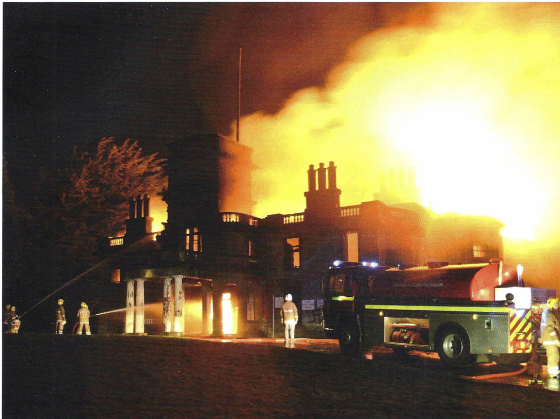
The Grade B listed Larbert House in Stirlingshire, which had been derelict for several years, was badly damaged by a fire in 2006. Designed by David Hamilton, the house was built for Sir Gilbert Stirling in 1822. (Photo: Central Scotland Fire and Rescue Service)
